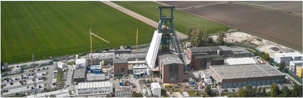
Fig. 5. The Konrad repository is an extension of an old iron mine. Source: BGE.
