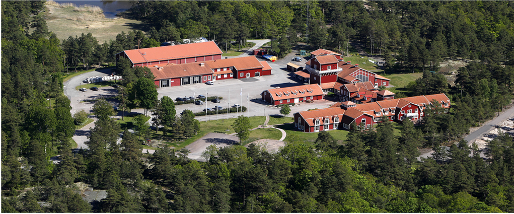
Fig. 14. The Äspö Hard Rock Laboratory surface buildings contain an exhibition building and are designed to blend into the surroundings. Source: courtesy of SKB.
